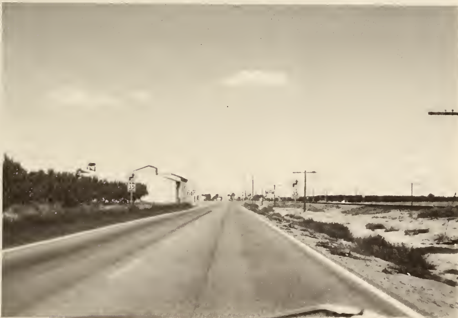
Figure 63 Roadside Clutter (Location 2)
